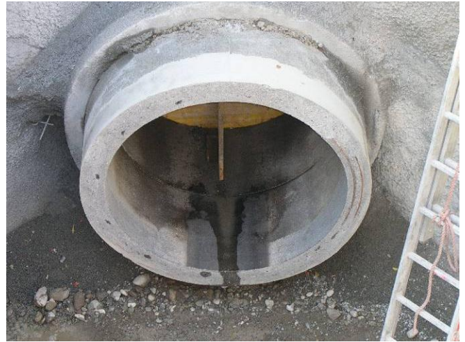
Rough pipe end cutting
