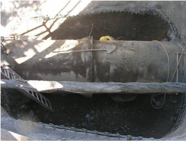
Before bell and spigot cutting
